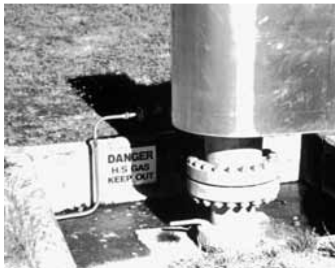
Figure 8.3 A sign warning of the potential danger posed by hydrogen sulfide in a well-head pit at Wairakei geothermal field in New Zealand
